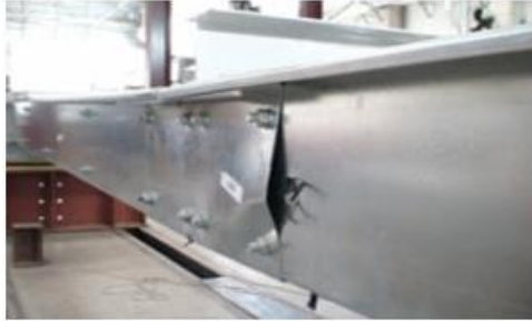
Figure 13: Failure mechanism at the end of the sleeve ZC83-L63
